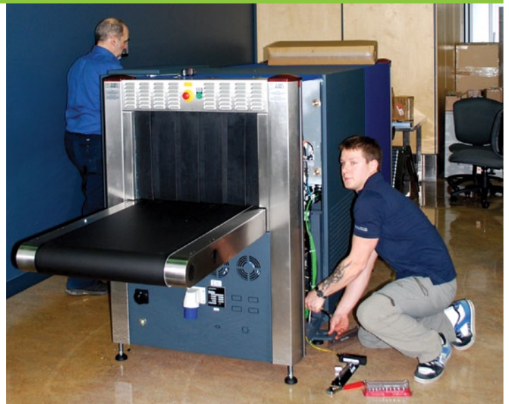
New X-ray machine being installed in pre-board screening.
